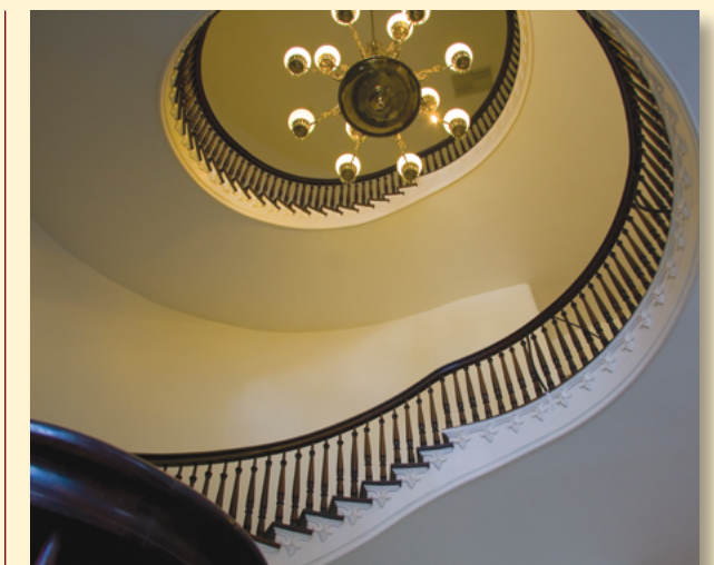
Above: This is one of the freestanding spiral staircases of the Alabama State Capitol. It is believed that Horace King built these beautiful stairs.
